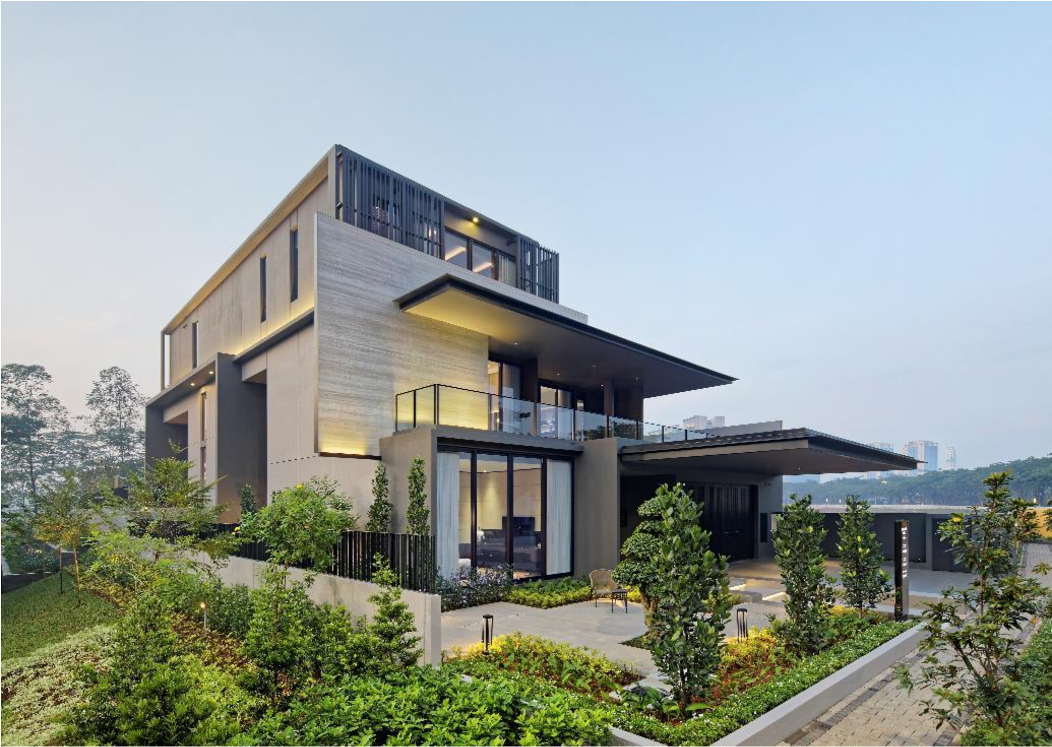
FACADE HADAP INTERNAL BOULEVARD
